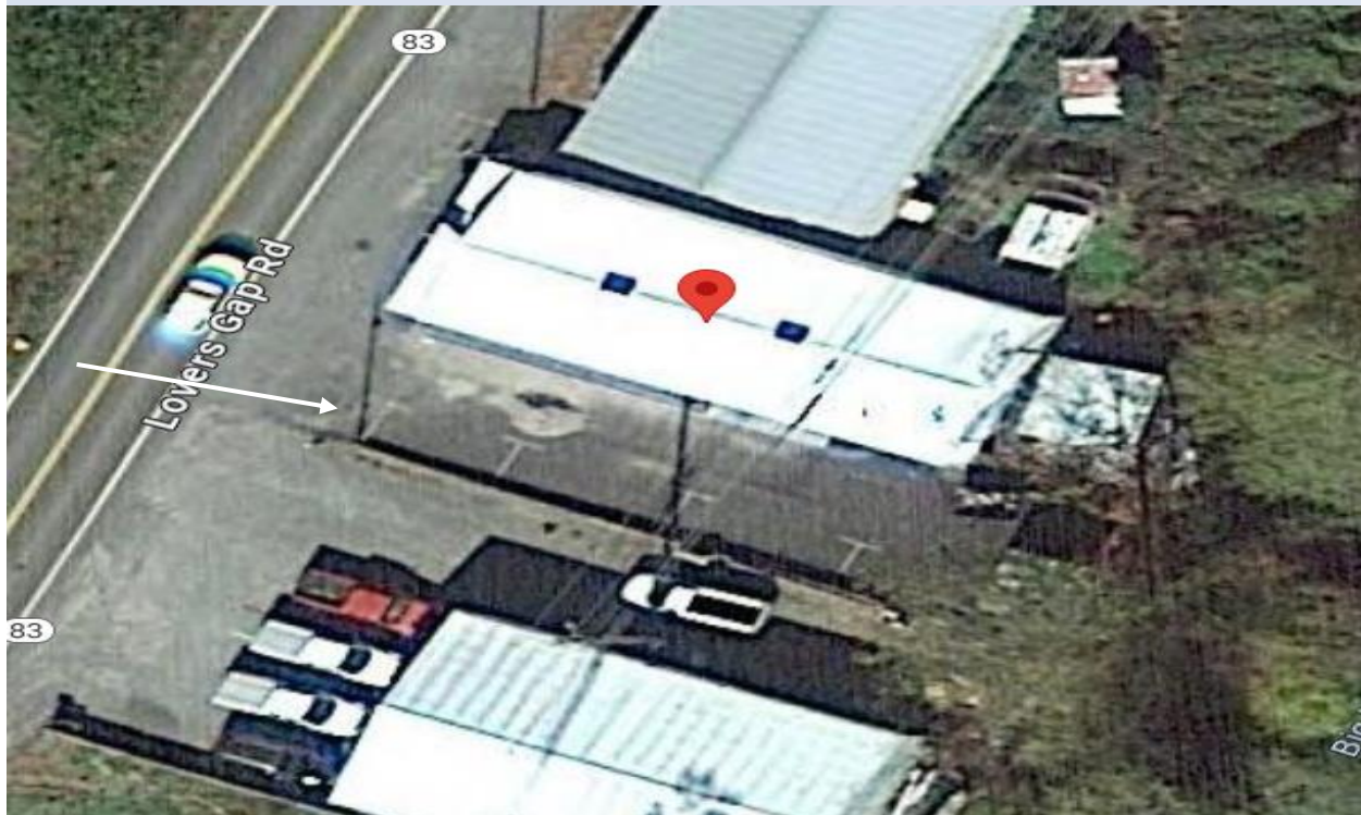
Parking lot between 2559 Lovers Gap Road and 2571 Lovers Gap Road
