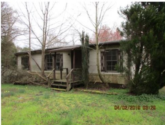
Main Structure Photo
