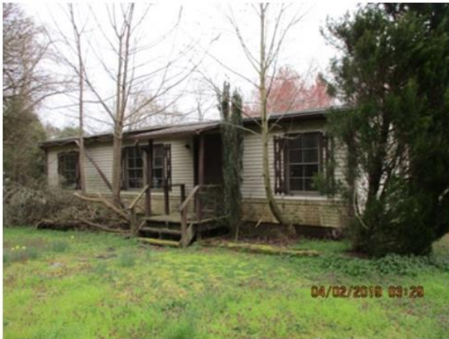
Main Structure Photo
